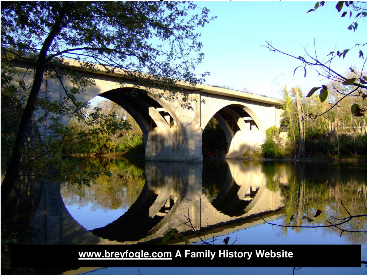
State Route 161 crossing the Scioto River, near Dublin, Ohio
