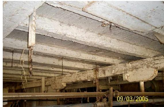
As we entered the barn from the farmyard, the ceiling appears to be original, which he indicated it was. The support beams were all hand-hewn timbers, perhaps cut by George Breyfogle, Sr. when the barn was constructed (1831).
